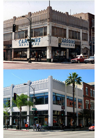
Figure 3.1.2 - A dilapidated building in Old Pasadena in the 1980s (above) and the same building now (below).
