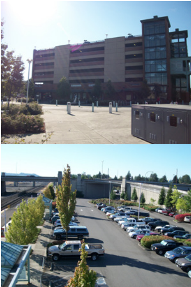
Figure 2.2.1 - The Auburn Transit Center garage (above) and surface parking lots (bottom) are already at capacity.
