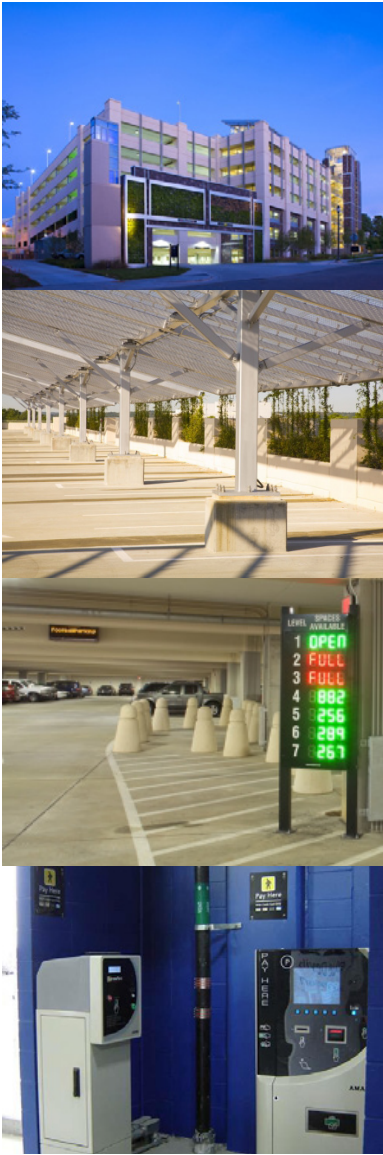
Figure 3.2.4 - The Duke University Research Drive Parking Garage features (top to bottom) vegetated rooftop canopies, space availability display boards, and pay stations prior to exiting.
